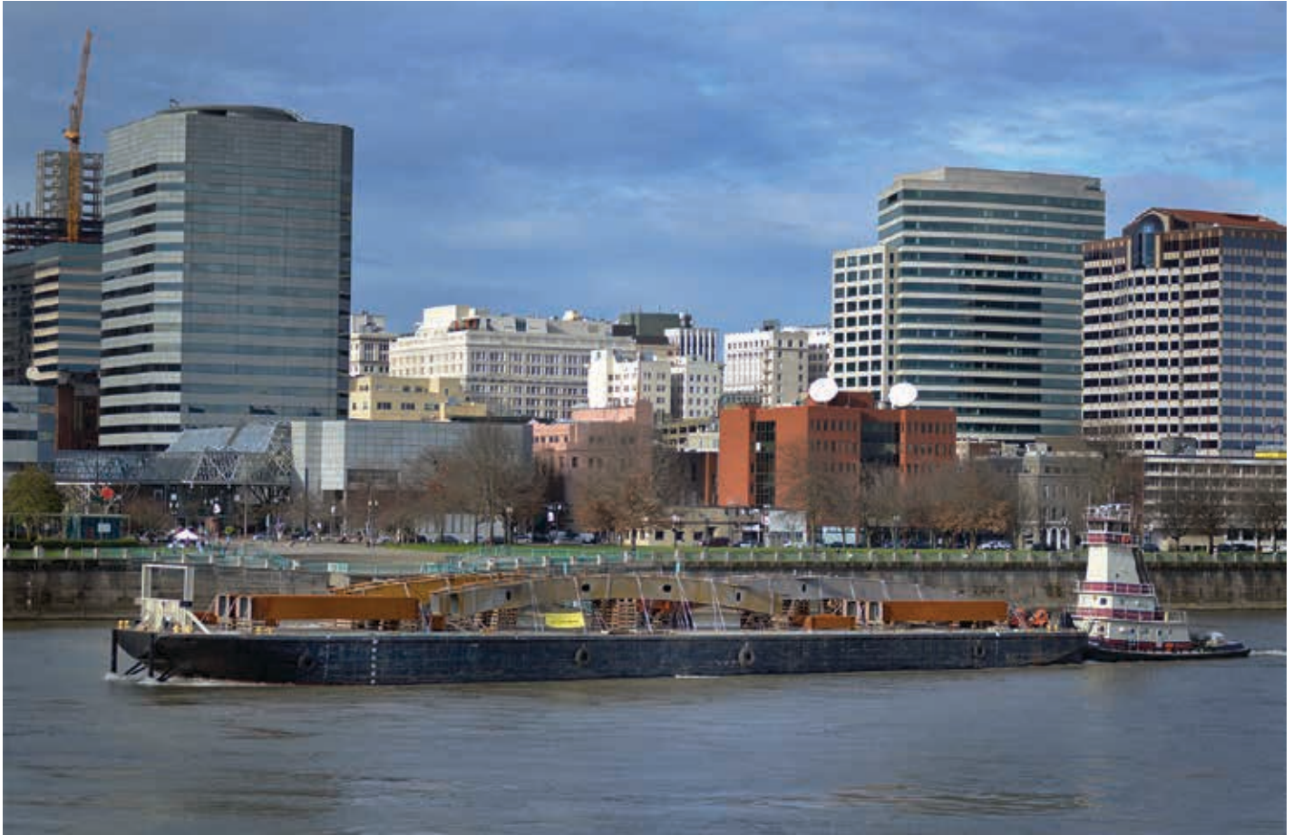
Barge carries segments for first two steel arch spans past downtown, December 2014
