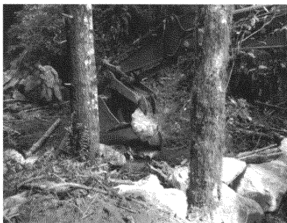
Heavy equipment carefully places boulders in the stream channel to improve salmon habitat.
