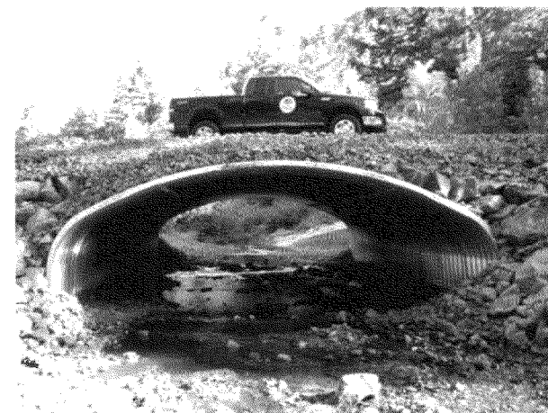
A new culvert on Maxfield Creek in the Luckiamute River Watershed.
