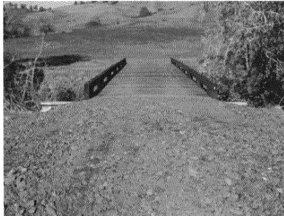
One of three railcar bridges used to prevent stream bank erosion from cattle crossings.
