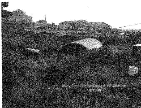
An open bottom arch culvert will create better fish passage on Riley Creek.
