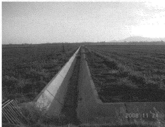
Concrete irrigation ditch installed to reduce sediment loading in the Lower Owyhee River.
