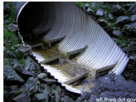
Culvert baffles
