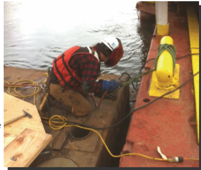
Female pile buck apprentice welds pile.
