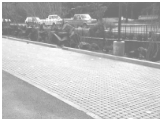
Pervious paving surface, Washington County, Oregon
