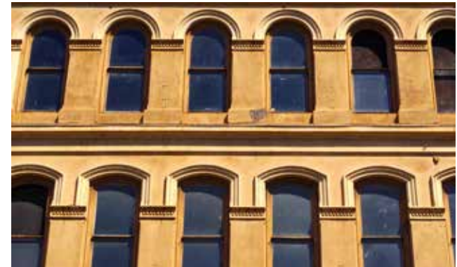
Narrow arched windows with hood molds
