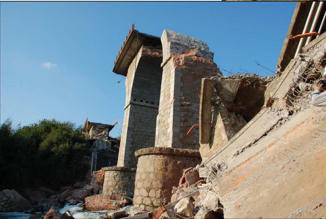
2010 Chili Earthquake Under-Reinforced Pier Failure
