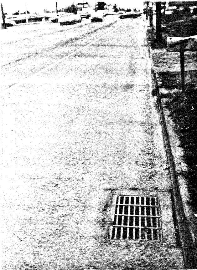
All parallel bar drainage grates located on County roads shall have steel cross straps welded perpendicular to the parallel bars. This will prevent bicycle wheels from dropping into the grate, potentially resulting in damage to the bicycle and injury to the rider.
