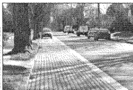
Pervious Paving Within Parking Lane
