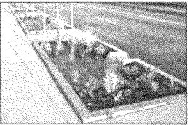
Vegetated Swale for Infiltration of Street Run-off
