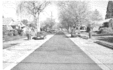
On SE 21st Avenue at Rex Street, permeable pavements allows water to go through the street surface and into the ground. It is the first use of this type of permeable paving material on a public street in Portland, although similar materials are used locally in parking lots and private driveways.
