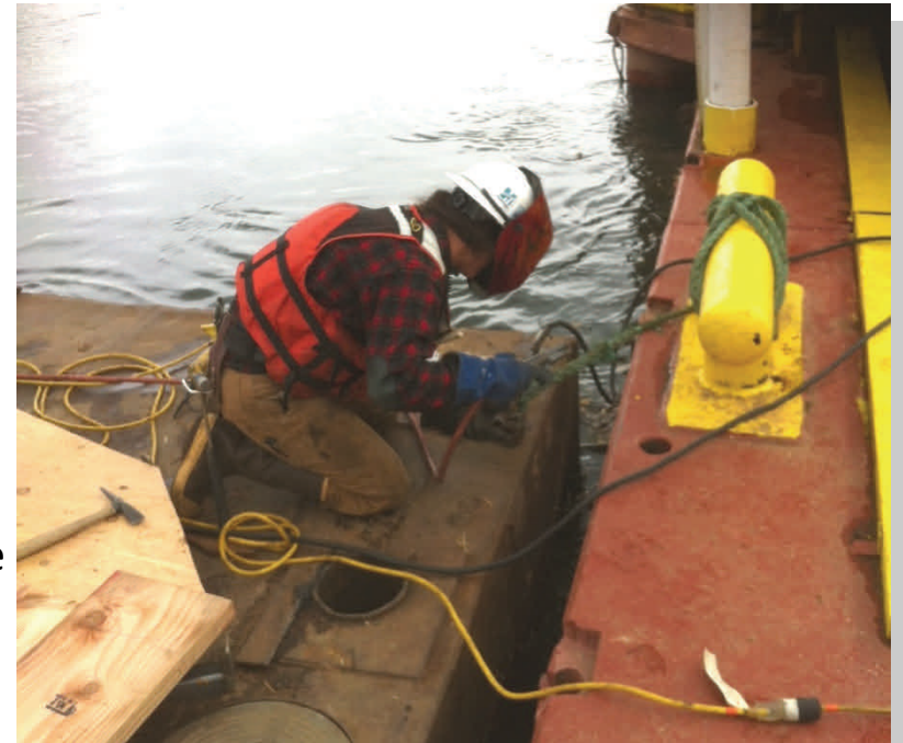
Female pile buck apprentice welds pile.
