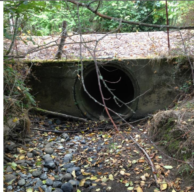
Above: 262 nd St. culvert, upstream end. Inlet is perched.
