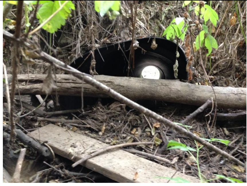
Above: Springwater culvert, upstream end. Steep slope & physical deformation.
