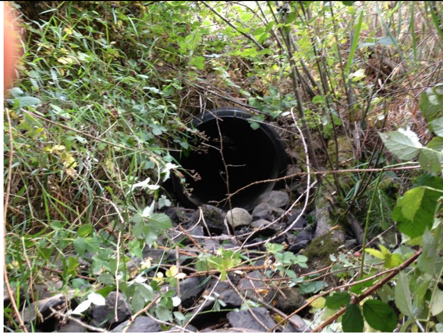
Above: Undersized Springwater Trail culvert, downstream end.
