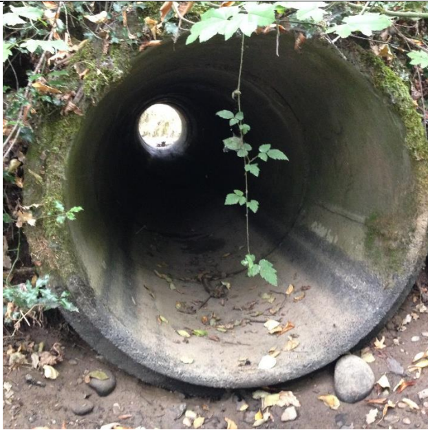
Above: 262 nd St. culvert, downstream end. Culvert's slope is a velocity barrier.
