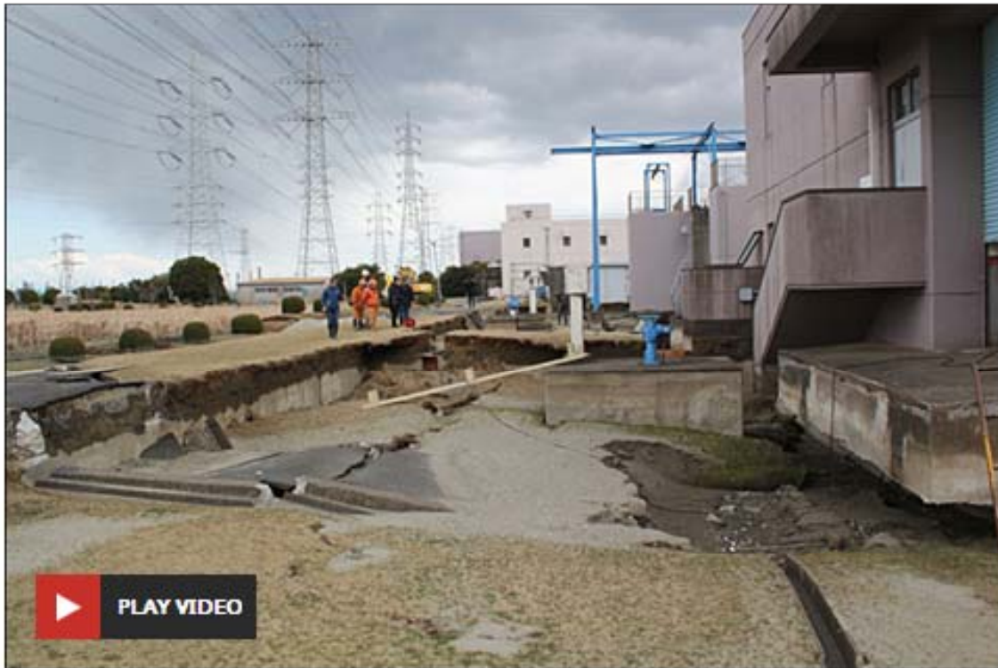
Liquefaction in the recent subduction zone earthquakes in Japan caused entire buildings to sink several feet lower than they had been previously. (Photo by Scott Ashford, courtesy of Oregon State University)
