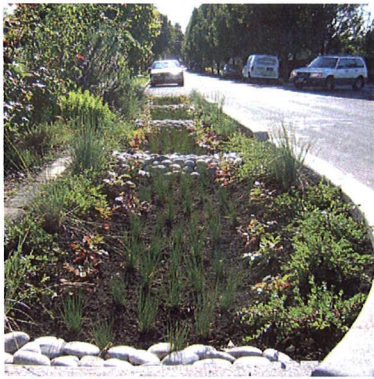
Designs showing stormwater treated naturally by soil and plants, instead of running into the sewer systems or polluting the river.
