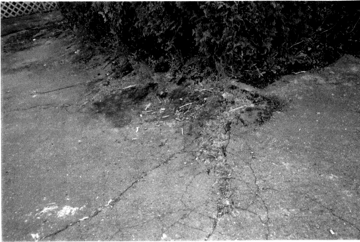
Surface roots in parking lot raising and cracking asphalt Bigleaf maple ( Acer macrophyllum ) Hillsdale Library
