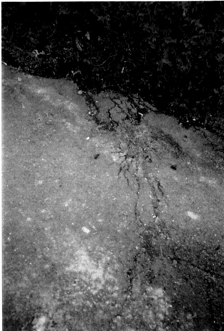
Surface roots in parking lot raising and cracking asphalt Bigleaf maple ( Acer macrophyllum ) Hillsdale Library
